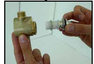
6 - remove and replace the cartridge
