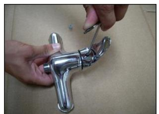
2 - loosen the screw of the handle
